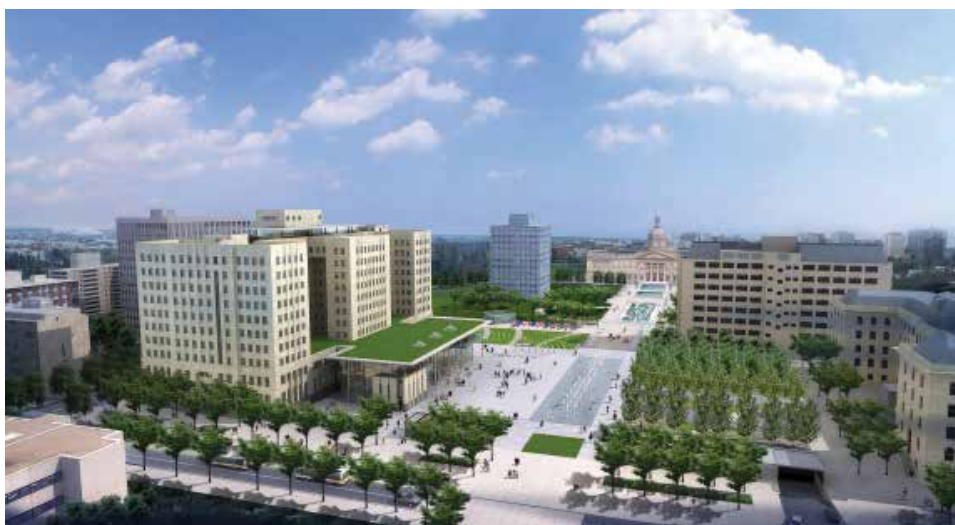
Aerial view (concept) of the Federal Building, Edmonton
