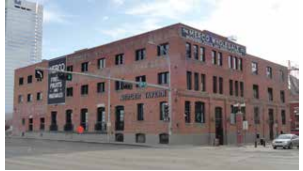
Mercer Building Edmonton
