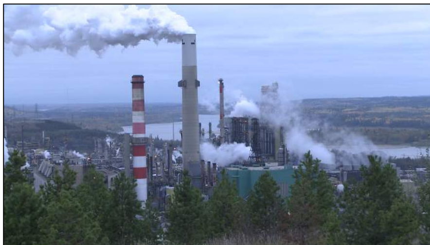
FIG 2.1. The Athabasca Oil Sands in operation (Suncor site)
